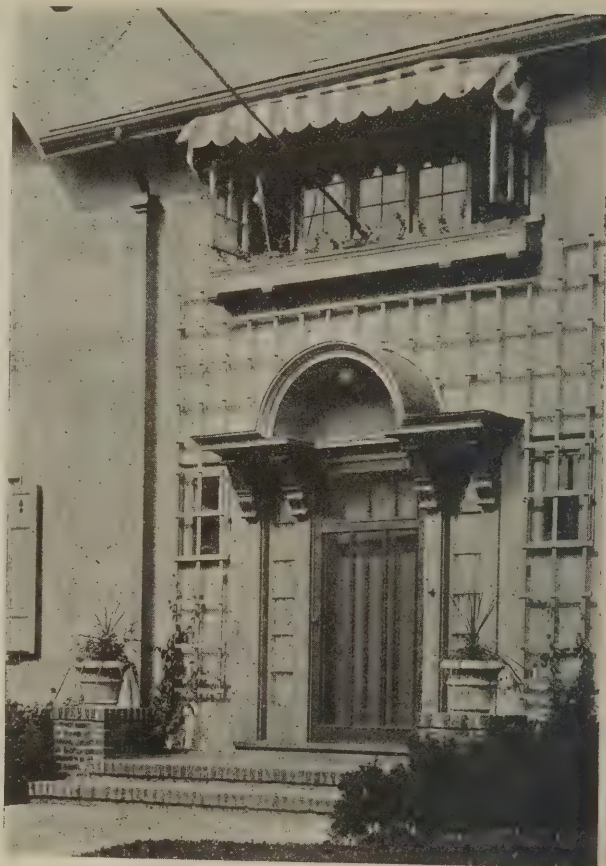
Shows a well carried out decorative treatment of a doorway. The correct lines of door and hood are well supplemented by the lattice and structural window boxes. Notice that the lines of screen door and the general form are in good keeping
